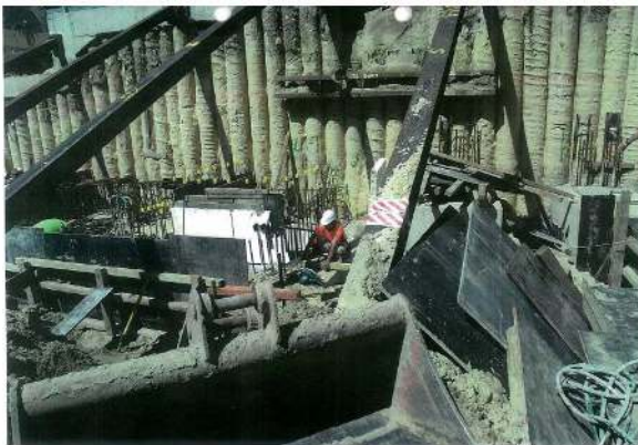
Figure L: Undated Photograph of Lift Shaft Excavation in Front of Waler Beam
