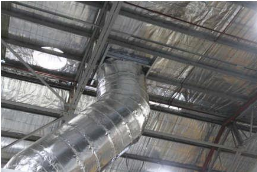
Photograph 4 - Northern flue roof penetration from the interior showing cut purlin and trimming purlins.
