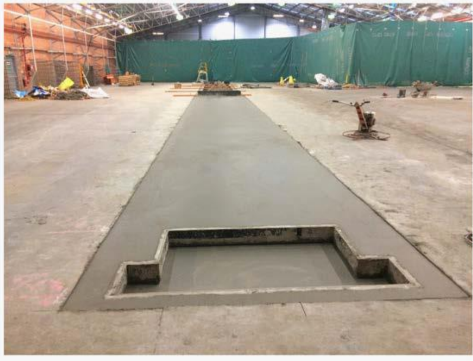
Photograph 3 - Freshly poured slab with finishing works in progress.
