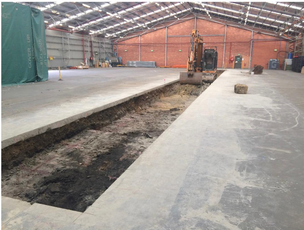
Photograph 2 - Slab cut out and excavation works in progress in 2017.
