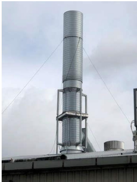
Photograph 6 - Southern flue with bracing frame/damper.
