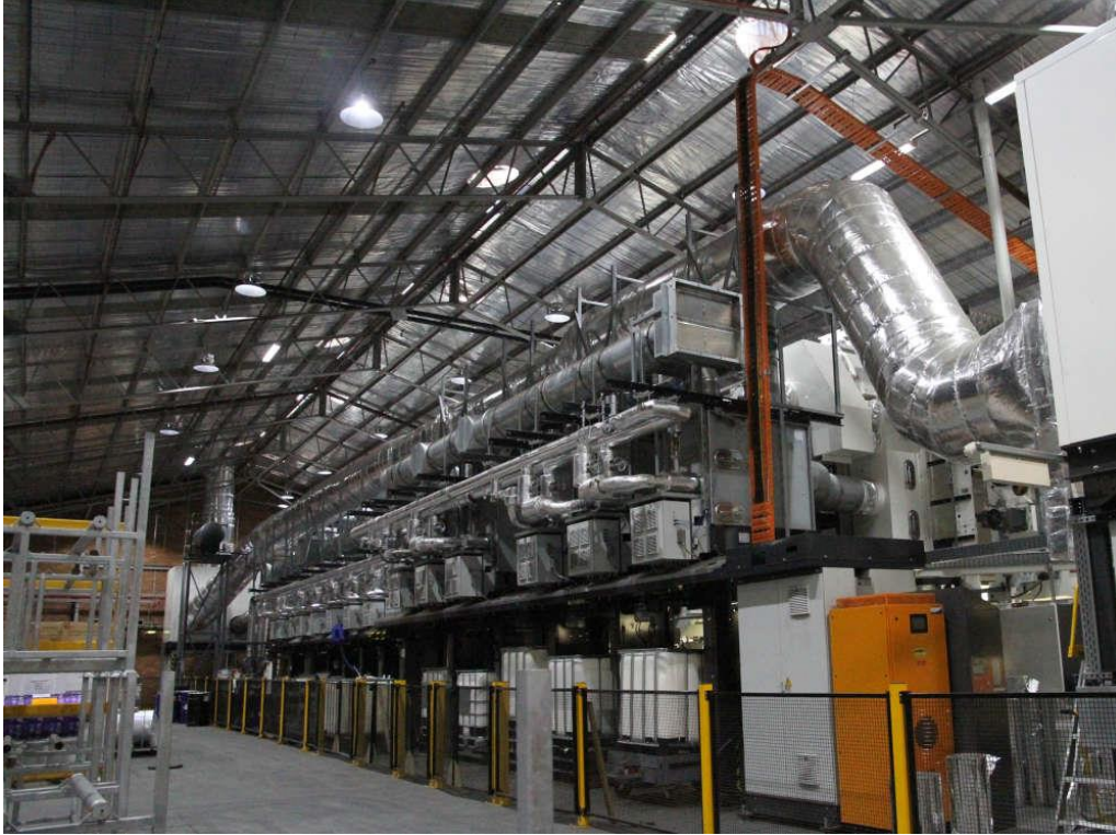
Photograph 1 - General view of interior of the building showing steel trusses, purlins and installed printing plant with southern flue at far end.
